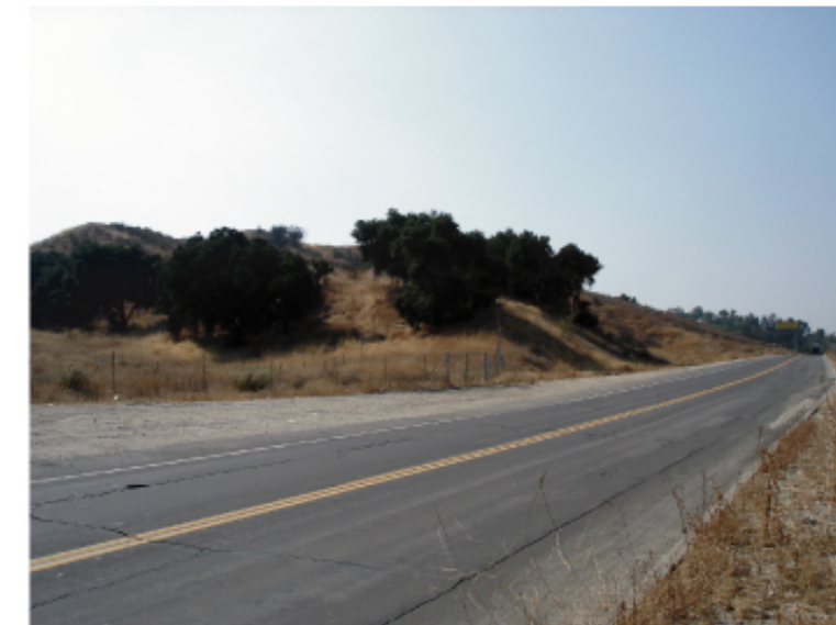
Site Photograph - Existing Condition
